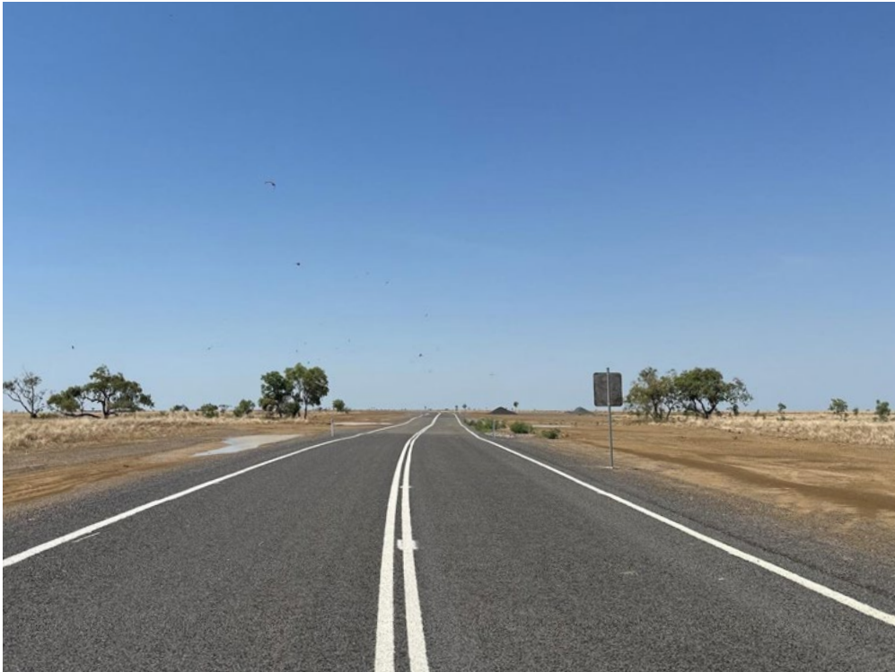
Image: Courtesy of the Department of Transport and Main Roads — Queensland Richmond-Winton Road upgrade.
