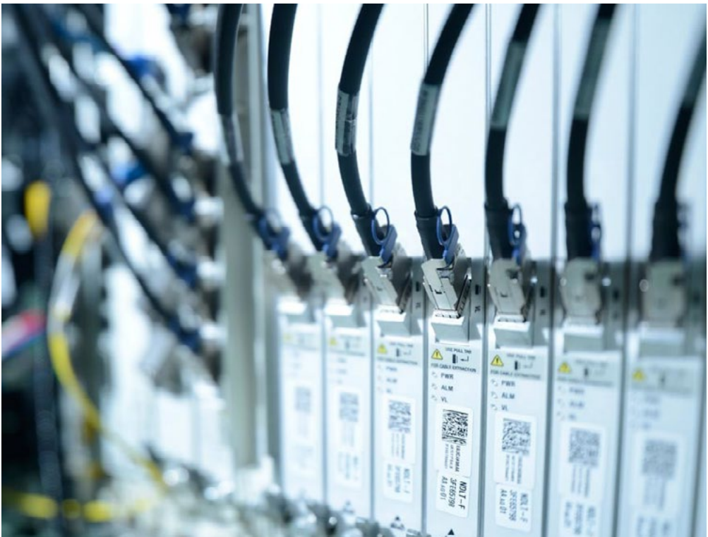
Image: NBN FTTN installation. Credit: DITRDCA
