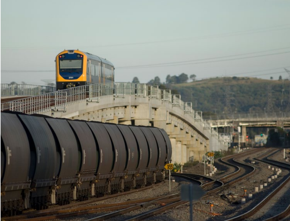
Image: Newcastle Rail, NSW. Credit: DITRDCA
