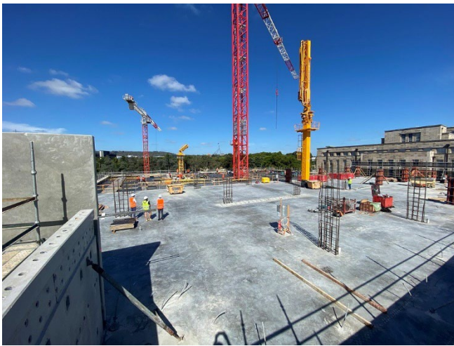
Level three of northern end of JGC Car Park site
