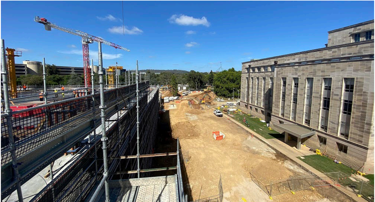
Northern end of JGC Car Park site
