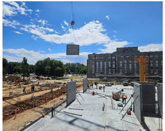
Installation of precast concrete
