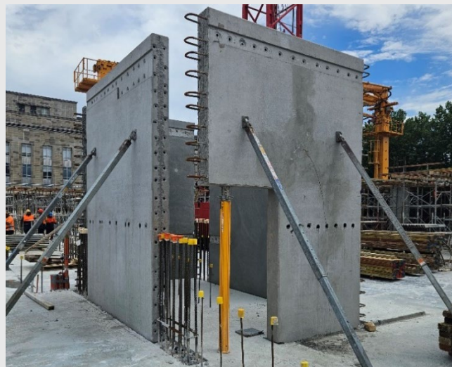
Precast concrete panels
